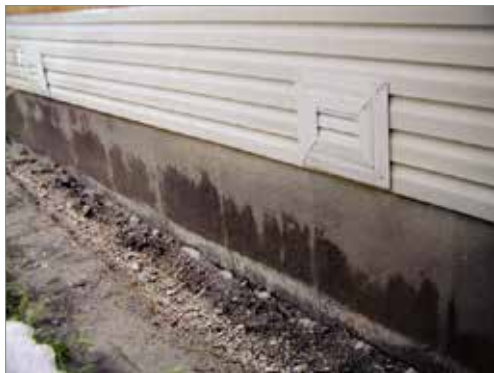
Moisture from the outside of a building from poor drainage can affect the slab inside and lead to floor failures.
