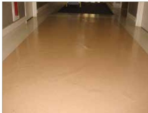
This sheet vinyl was installed in a 50-year-old hospital, and no moisture testing was done prior to installation. For reasons unknown, the previous tile floor did not exhibit any problems, but the new floor did. Moisture testing could have warned of this potential problem.
